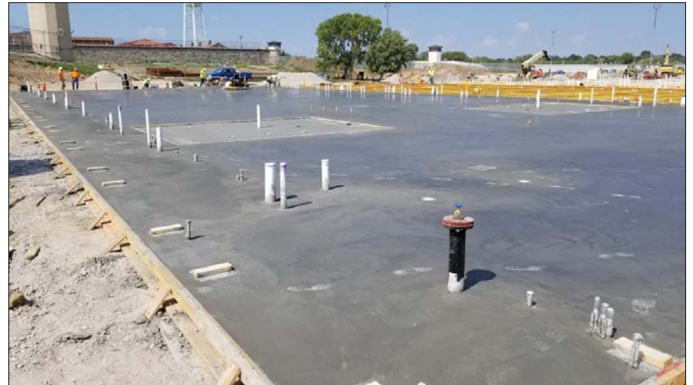
Building B Slab-On-Grade
