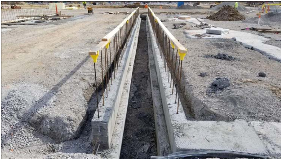
Support Building Footings
