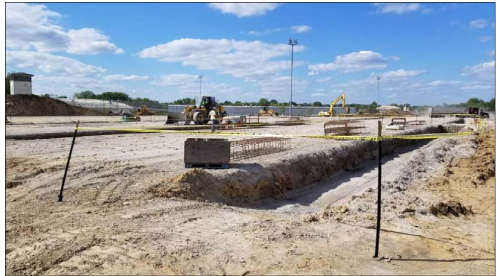
Building A Footing Excavation
