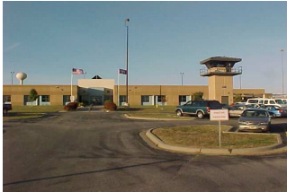
El Dorado Correctional Facility - Administration building
