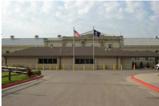
Hutchinson Correctional Facility
