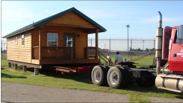
In conjunction with the Kansas Department of Wildlife and Parks, cabins built by inmates have proven to be popular among state park users as well as inmates who gain valuable construction experience.
